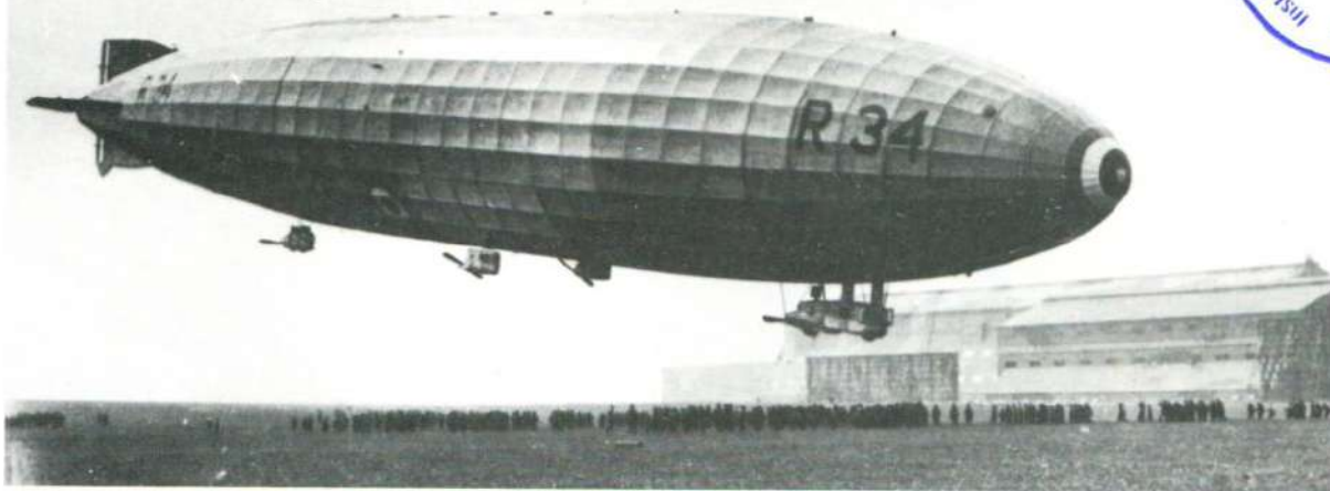
Back at East Fortune: note worn outer covering.
