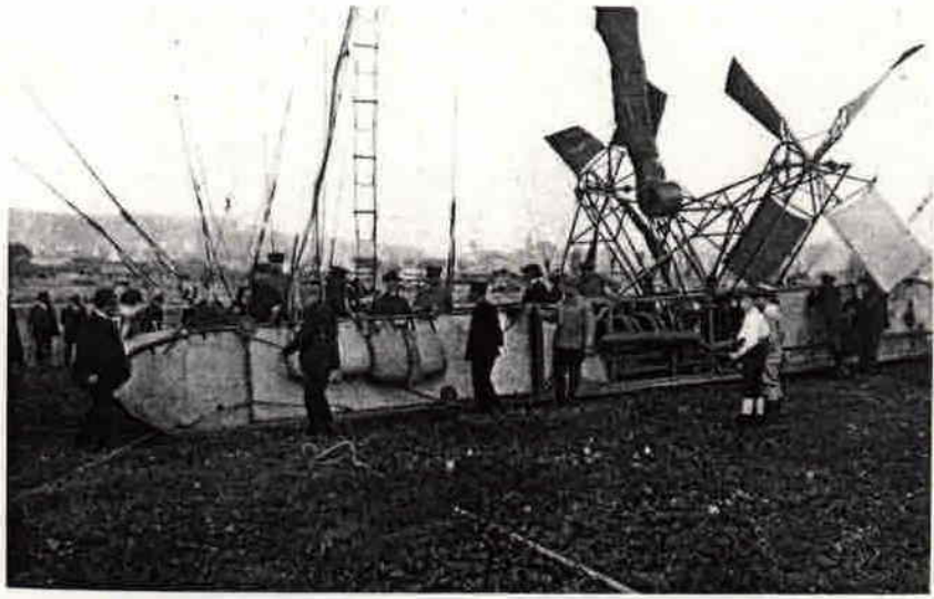
1.11. Gondola-framework of the Parseval PL VI. (Courtesy of the Swiss Transport Museum)
