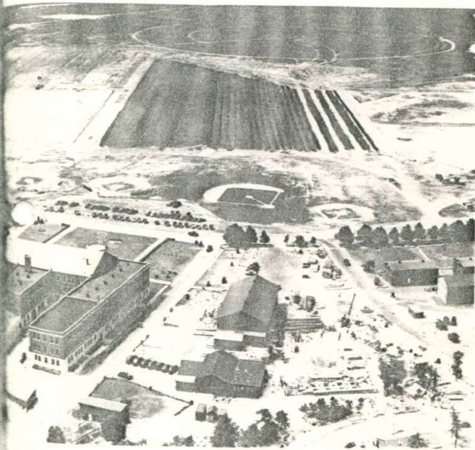
Paving of Mat 1 gets underway (top) at NAS Lakehurst, July 1942. Under the pressure of war, the grass landing field surrendered to the demands of intense air traffic and the need for a runway-like surface. It had become routine for the patrol airships to take off heavy like an airplane. (National Archives)
